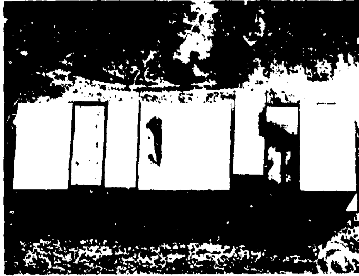
Figure 4.65 Post-Dogwood Olive, and -Pine, (Item 26) Station 3.1.1, aerial view. Pressure levels: Dogwood, 12 psi; Olive, 8.4 psi; and Pine, 13 psi.
